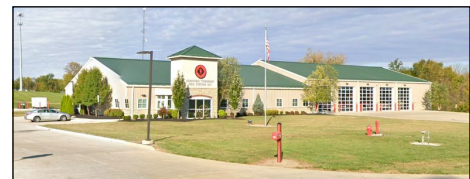
Concord Township Fire Station
